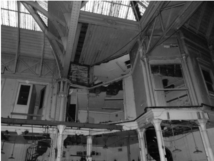
Rotten timber flooring and wall cladding
