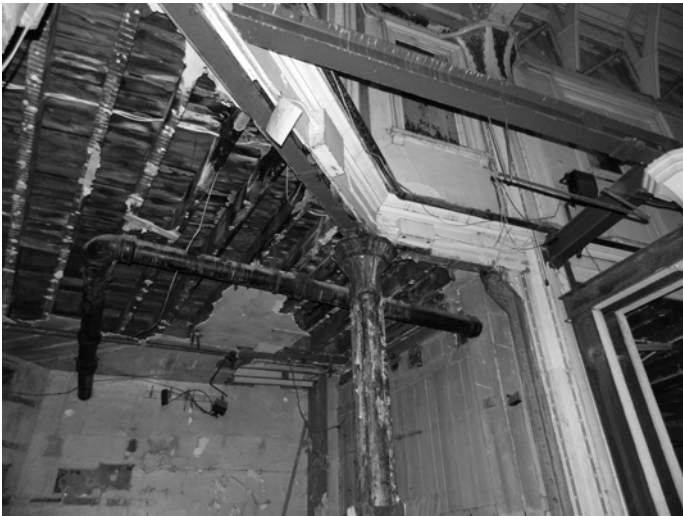
Corroded cast iron columns
